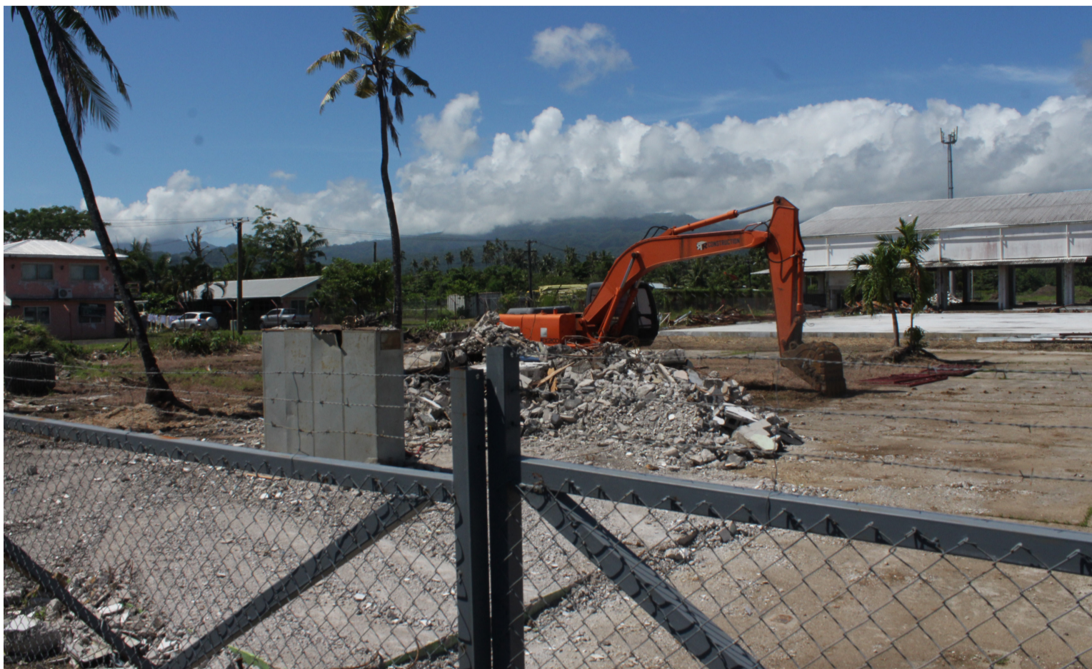
Landscaping work continues at Apia Park.
