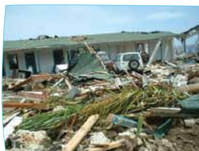
Damage from Tropical Cyclone Heta, January 2004.
