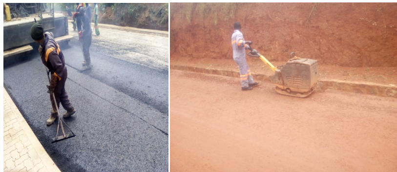
Figure 11. Lack of Protective equipment's like masks, helmet and gloves at Karama and Akagera Roads respectively during implementation on site.
