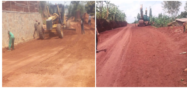
Figure 1. Lack of safety measures for site workers with construction equipment.
