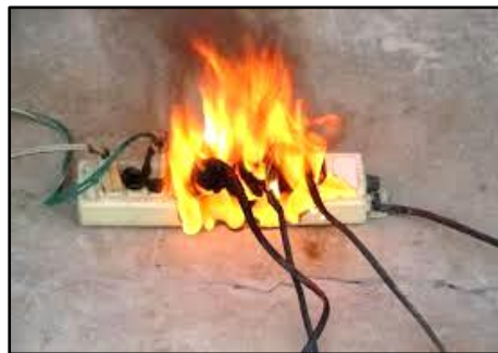
Figure 11. Multiple electricity base catch fire.
