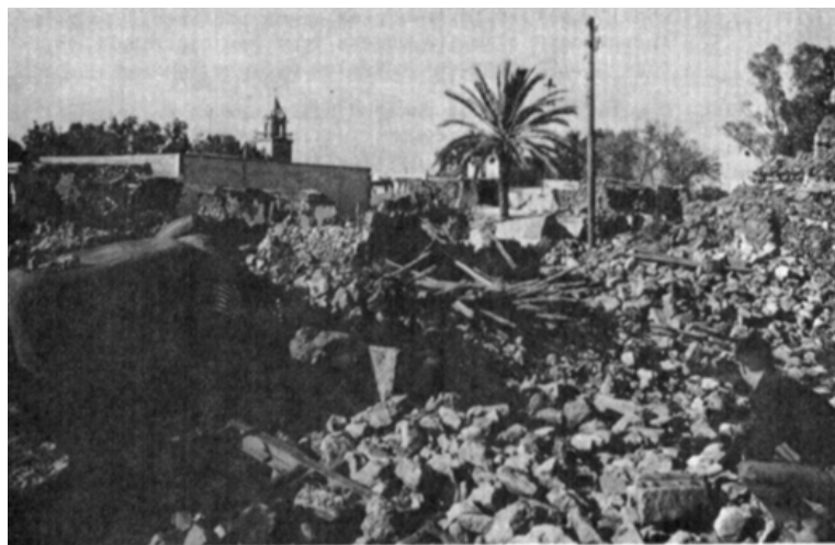
Figure 3. The heap of rubble stones in the popular housing area. In the center is the remainder of the fallen roof consisting of wooden rafters. Among the ruins, a building with girders and reinforced concrete columns remain standing though damaged [19].
