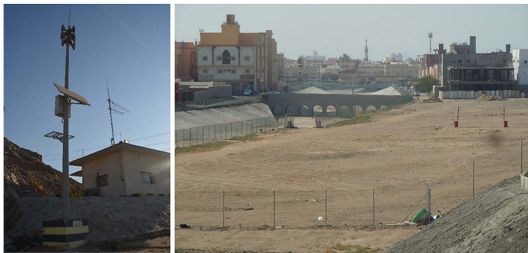
Figure 16. Buildings close to water canals (right). A dam's alarm system (left).
