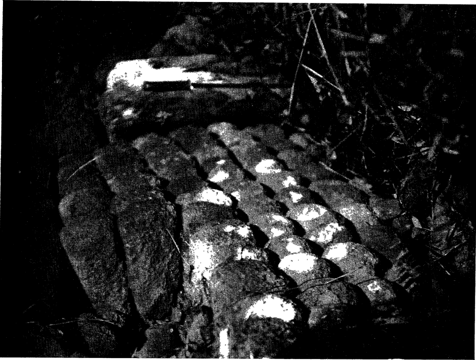
A.—MARAÉ HORORA, MOOREA ; SECTION OF BOUNDARY WALL. (LENGTH OF KNIFE, 1 FT. 9 IN.)
