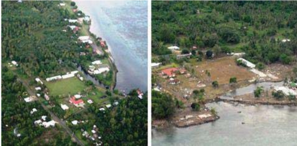
Figure 1: Aerial pictures of Poutasi before and after the Tsunami
