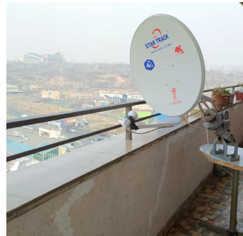
Figure 1. Ku-band, 60 cm dish antenna and LNB of ArtAr-HDF are installed on mechanical scanner at a height of 52 m from the ground in Yerevan and directed West, South-West to measure sky emission and solar emission during sunset.
