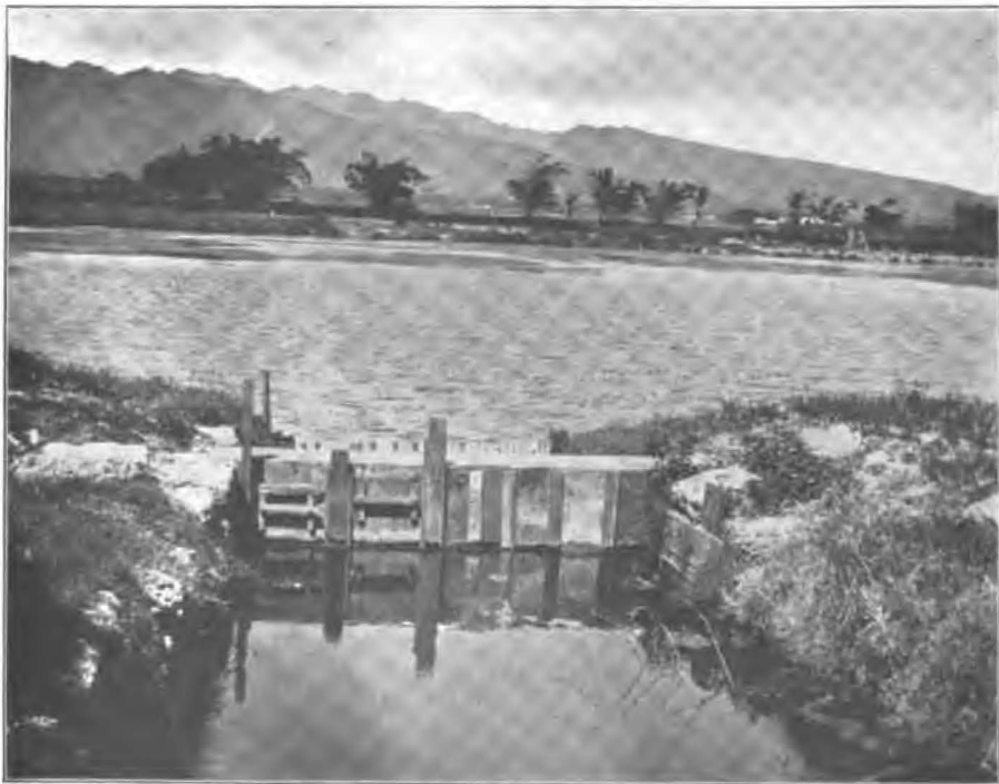
SLUICeway LEADING INTO INTERIOR FISH POND, WAIKIKI, OAHU.
