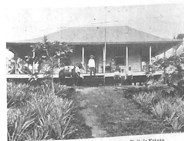
Residence of Overseer, Manga Station, Vailele Estate.
