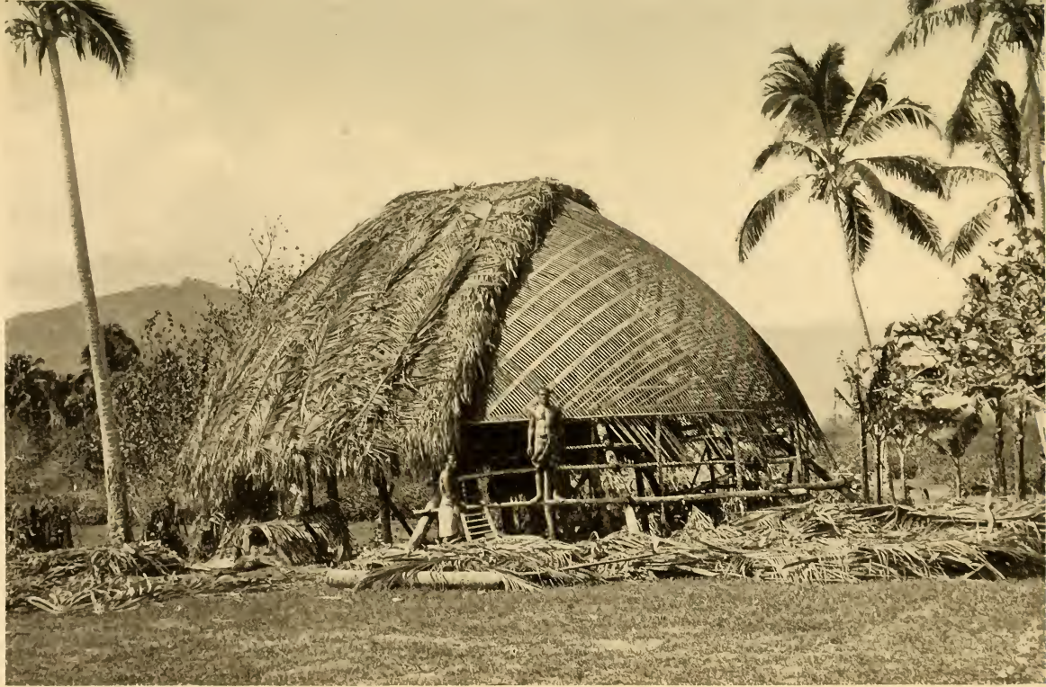
A Samoan house is merely a roof of thatch set up on posts
