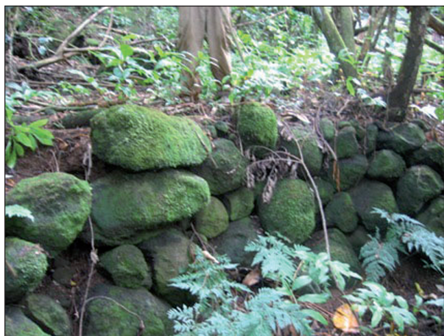
Figure 7. Stone retaining wall near the northern termination point of Feature 38.
