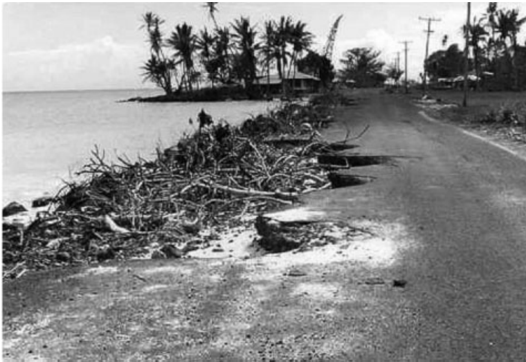
Figure 1. Coastal erosion affecting infrastructure, including the house in the background (photograph from Beca International)
